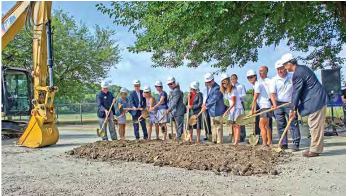
School district and city officials formally break ground Tuesday for construction of the new $4-million Lane Stadium project at Old River. When completed in the spring of 2017, the new stadium will house the track and field, lacrosse, field hockey, and soccer for Oakwood schools.
